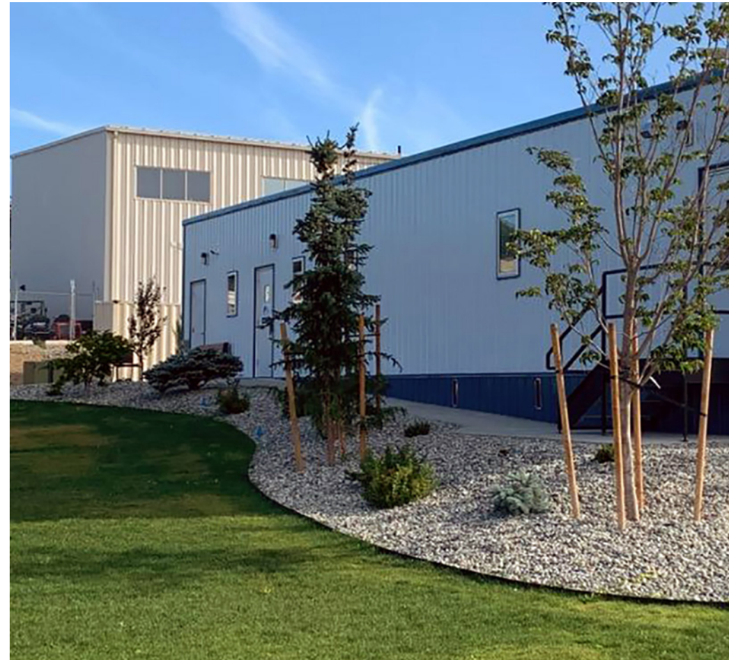
Eurofins Idaho Food Safety Laboratory. Built by Art's Way Scientific, Inc. & PSE Consulting Engineers Inc. First Place, Relocatable Modular Special Application.
