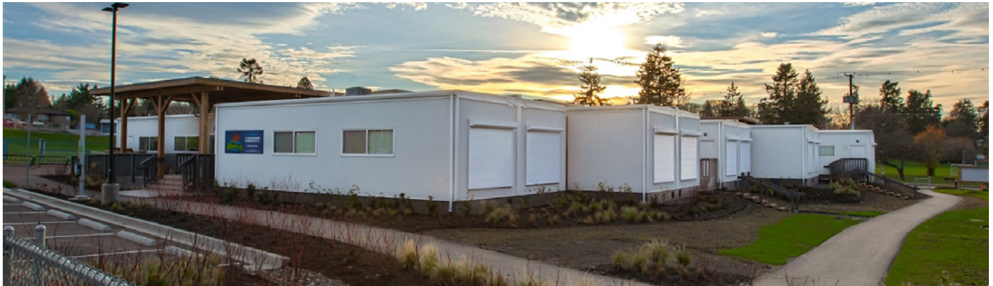
CSF Beausoleil School, Built by Fort Modular First Place, Relocatable Modular Education Over 10,000 Sq. Ft.
