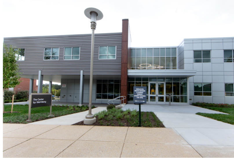
The Center for Well-Being, University of Maryland, Baltimore County (exterior) Built by MODLOGIQ & Whiting-Turner First Place, Permanent Modular Healthcare Over 10,000 Sq. Ft.
