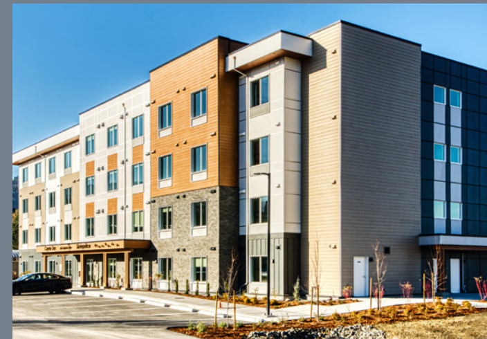
Cover Image: Thompson Rivers University housing. Built by NRB Modular Solutions with TechCanada Contracting Ltd. and S2 Architecture. Kamloops, BC, Canada.
