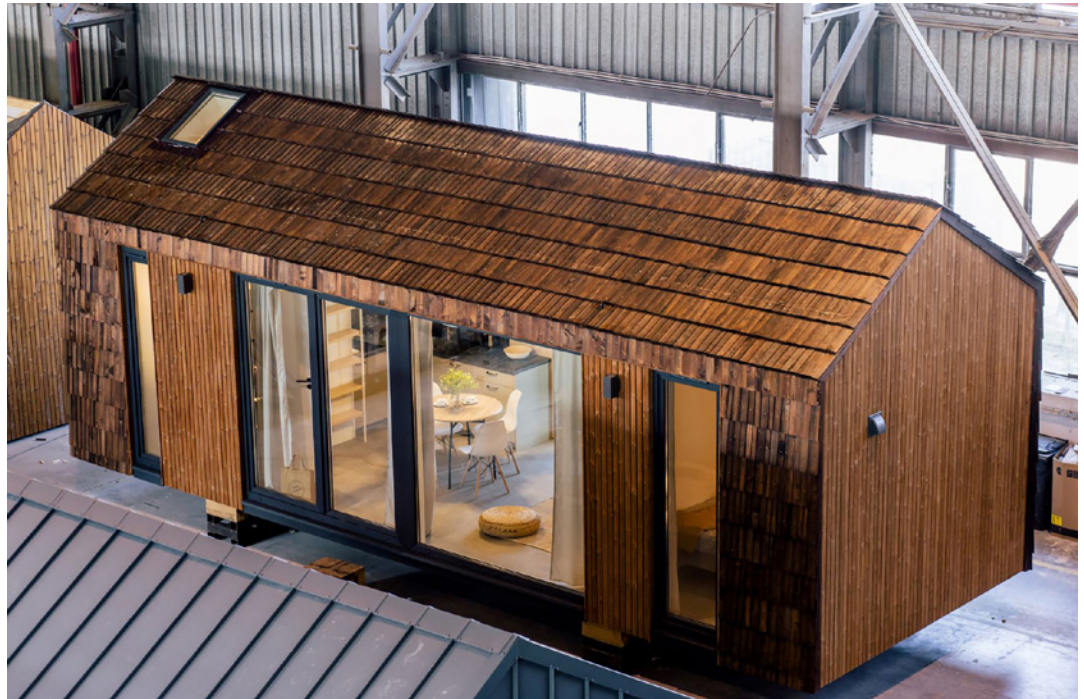
Smart House (exterior). Built by DMDmodular, Sp. z o.o.
