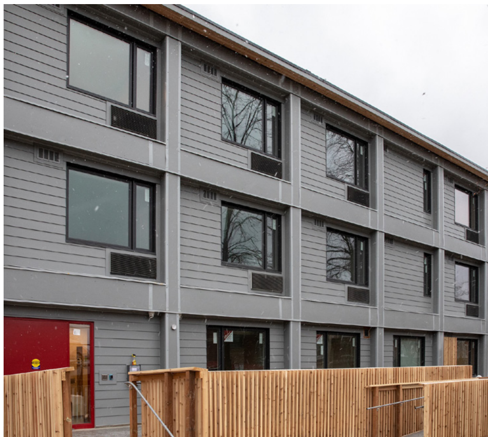
Recently-constructed Harrison Street supportive housing development in Toronto, built by NRB Modular Solutions.
