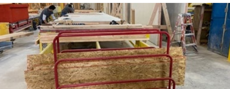
Figure 4: Reuse of Wood Framing in Factory
