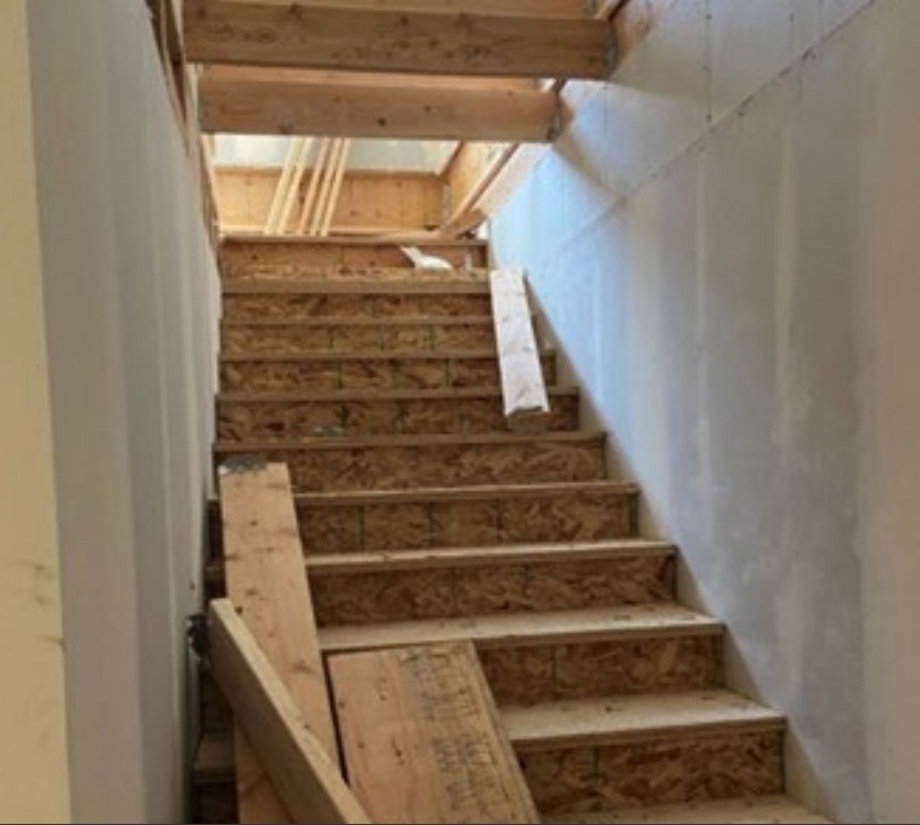
Figure 8: Adjoining Framing of Modules
