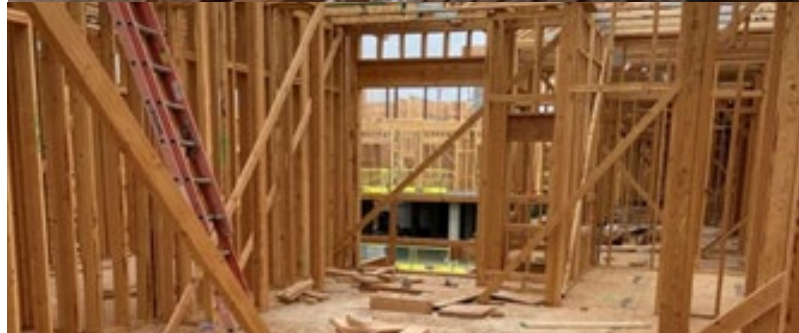
Figure 10 & 11: On-Site Wood Waste
