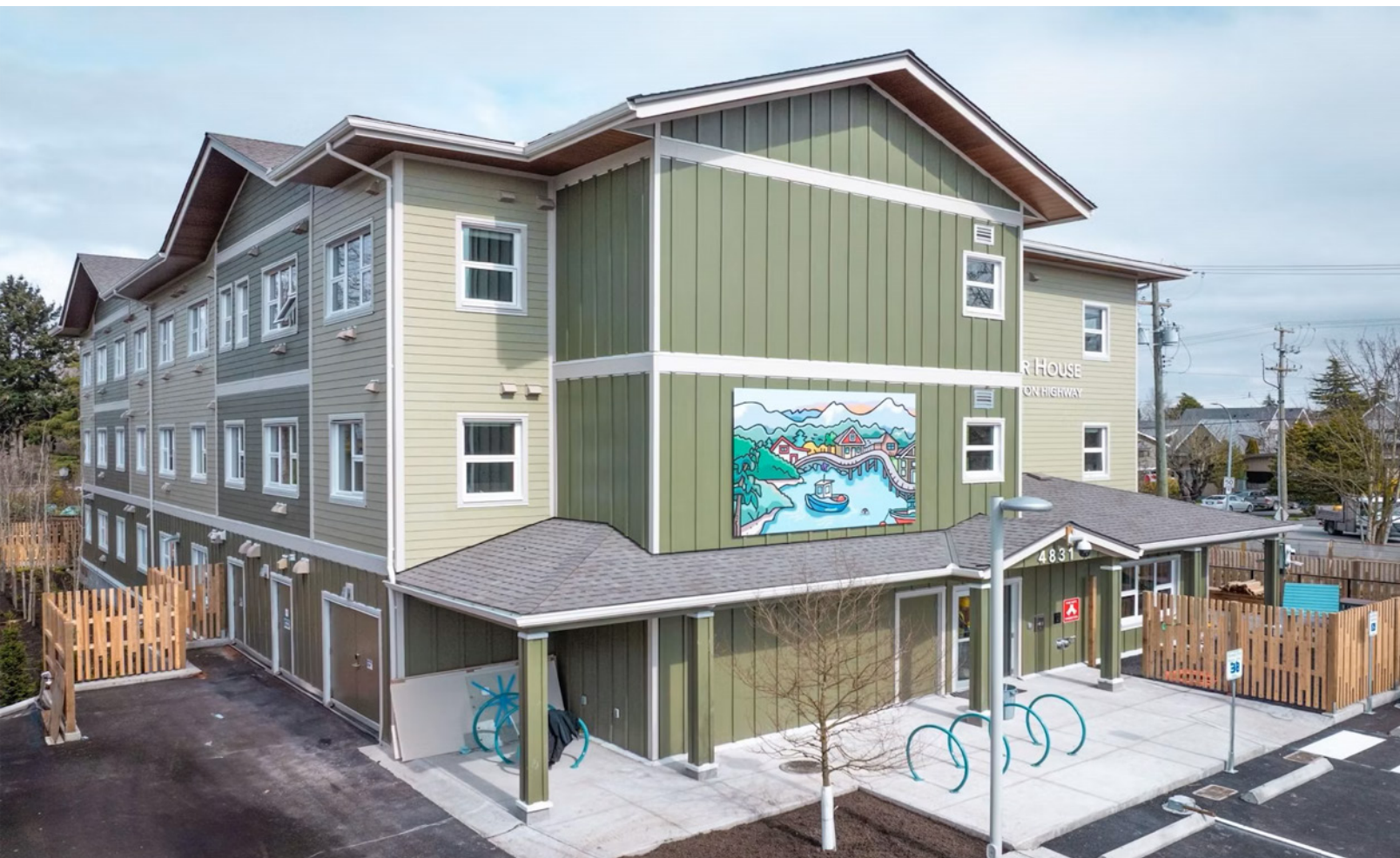
Steveston Hwy Affordable Housing, Richmond, BC. A 33-module, 20,750-sq. ft. permanent affordable housing complex built by ROC Modular with affiliate Buttcon Limited.
