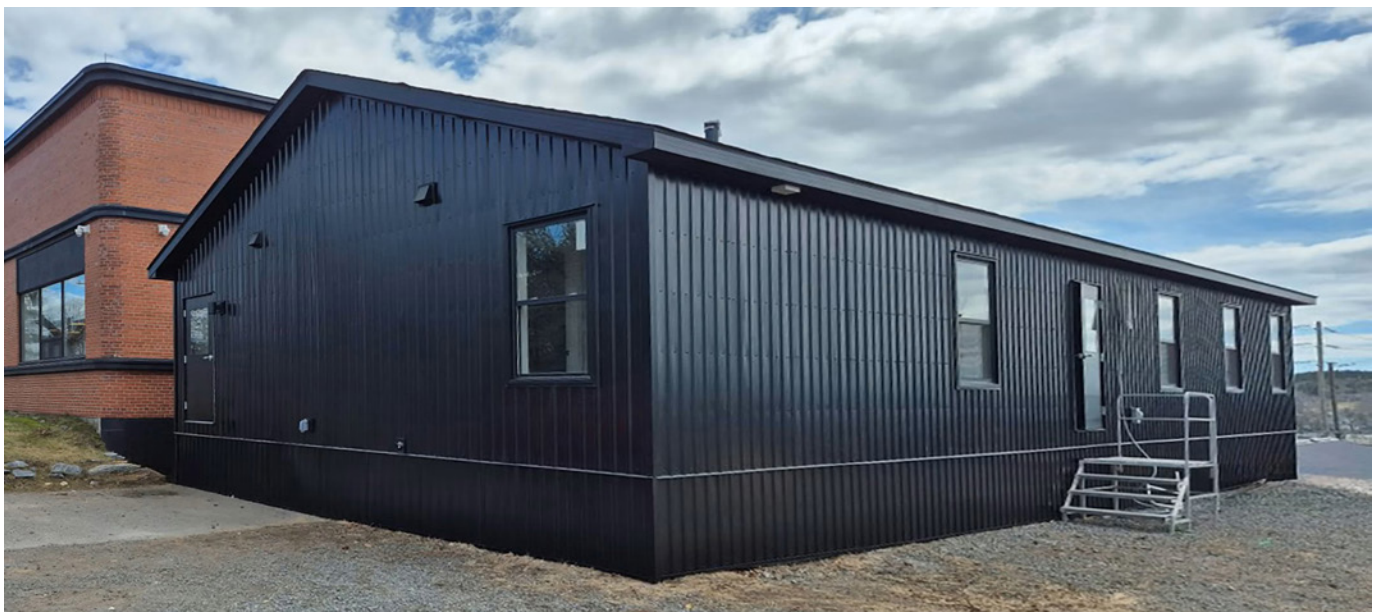
Saint John Museum - Staff Room, Saint John, NB. An 2-module, 1,740-sq. ft. staff gathering facility built by Kent Homes.
