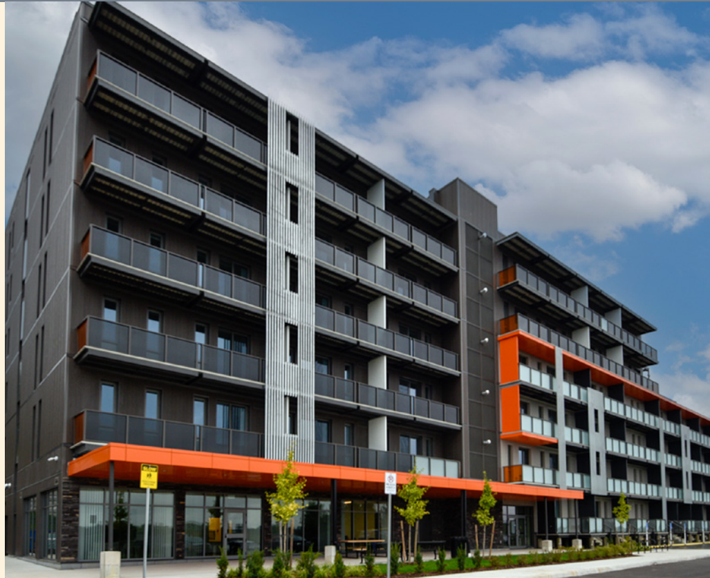
FUZE Woodstock, Woodstock, ON. A 183-module, 92,000-sq. ft. multifamily project designed by Skyhook Modular with affiliates Z Modular Holding Inc, Melloul Blamey Construction, Entuitive, and Quasar.
