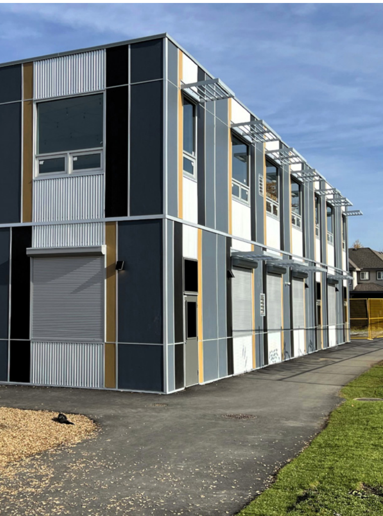
Lynn Fripps Two-Storey Permanent Modular Addition, Langley Twp, BC. An 18-module, 9,900-sq. ft. educational facility built by Fort Modular Inc.
