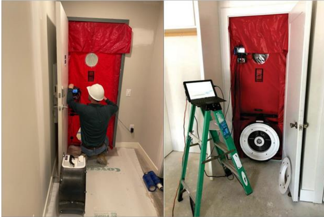
Figure 48. ANSI/RESNET/ICC 380-2019 envelope leakage test setup.
