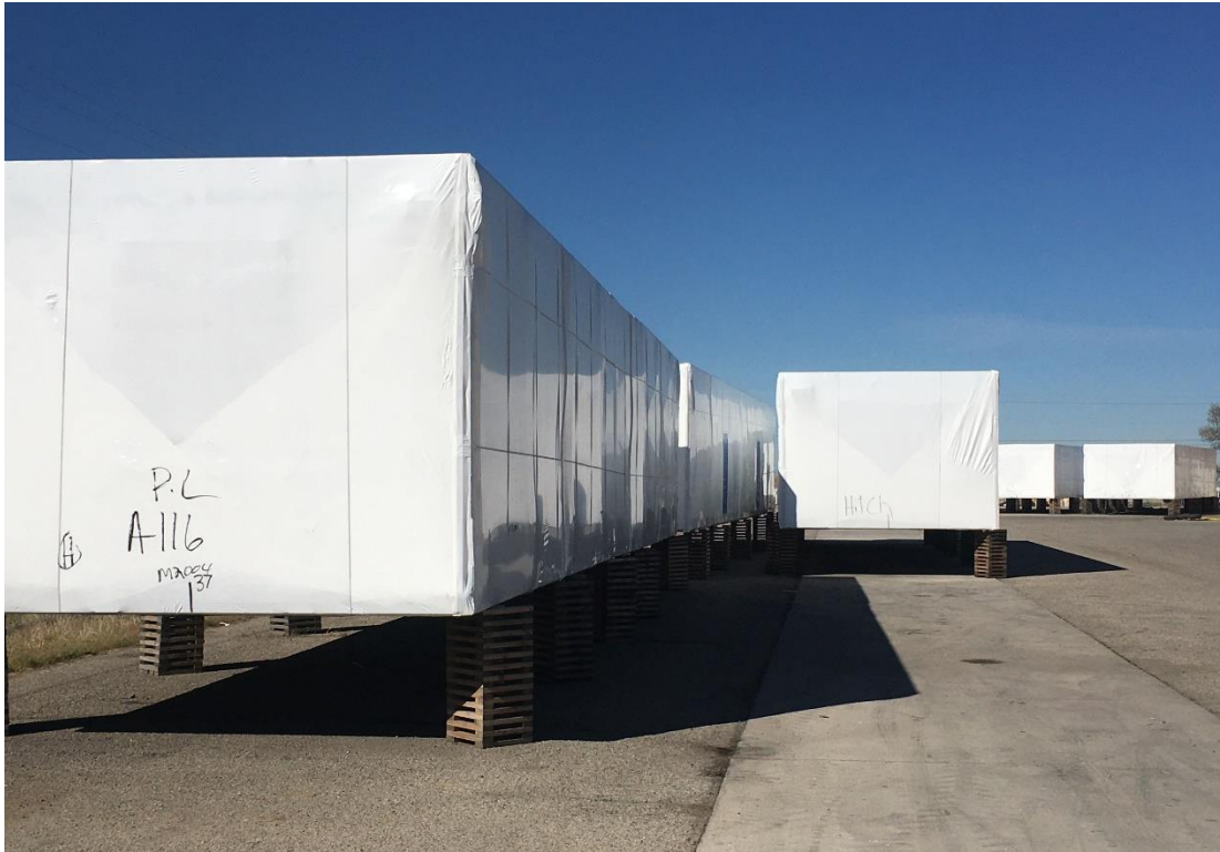
Figure 56. Offsite storage and staging area required for modular construction.
