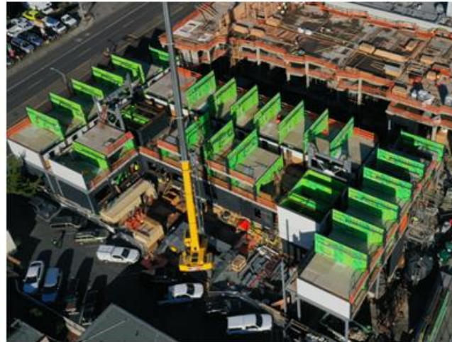
Figure 5. Volumetric and non-volumetric modular construction process.
