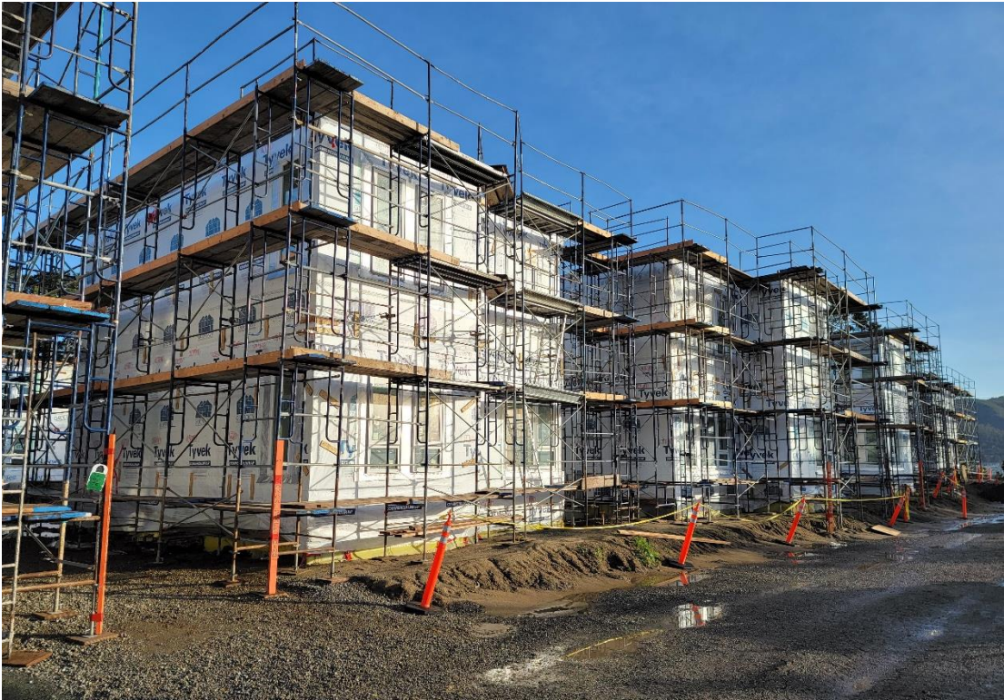
Figure 54. Onsite modular exterior finishes.
