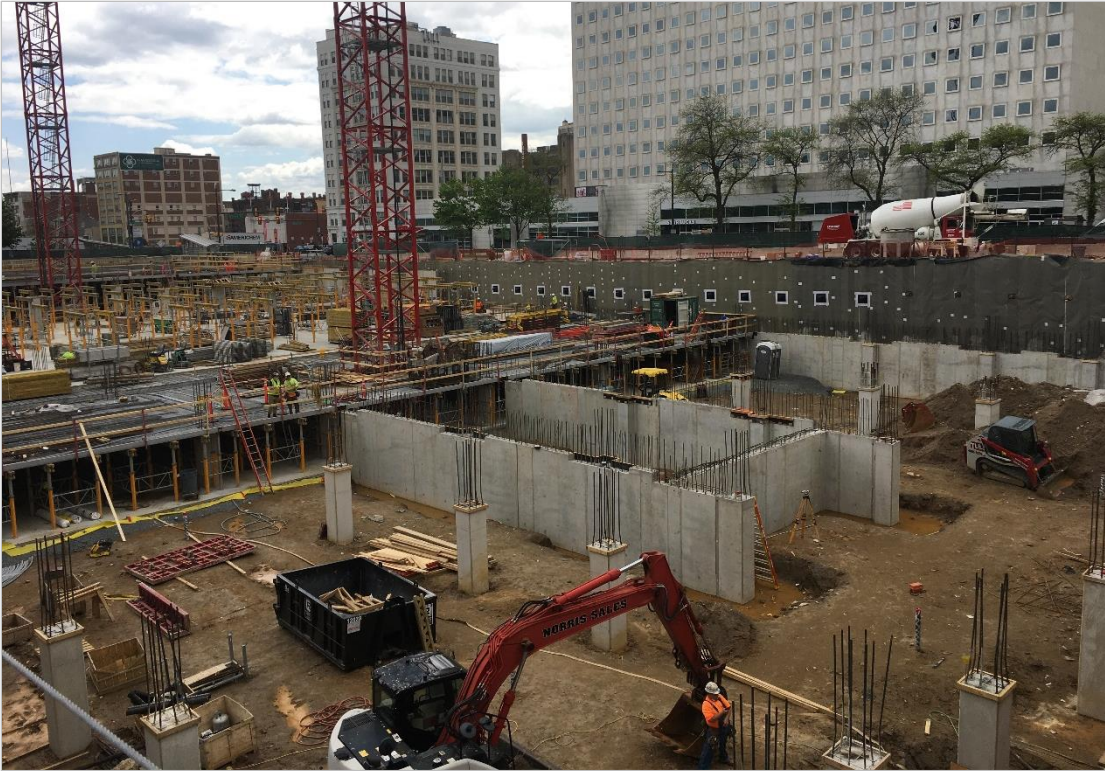
Figure 53. Onsite modular foundation construction.
