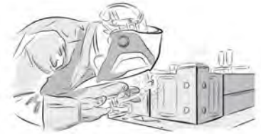
Fabricators weld the VectorBloc into place.
