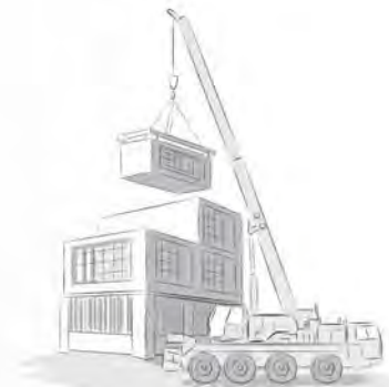
Modules easily stack on-site.
