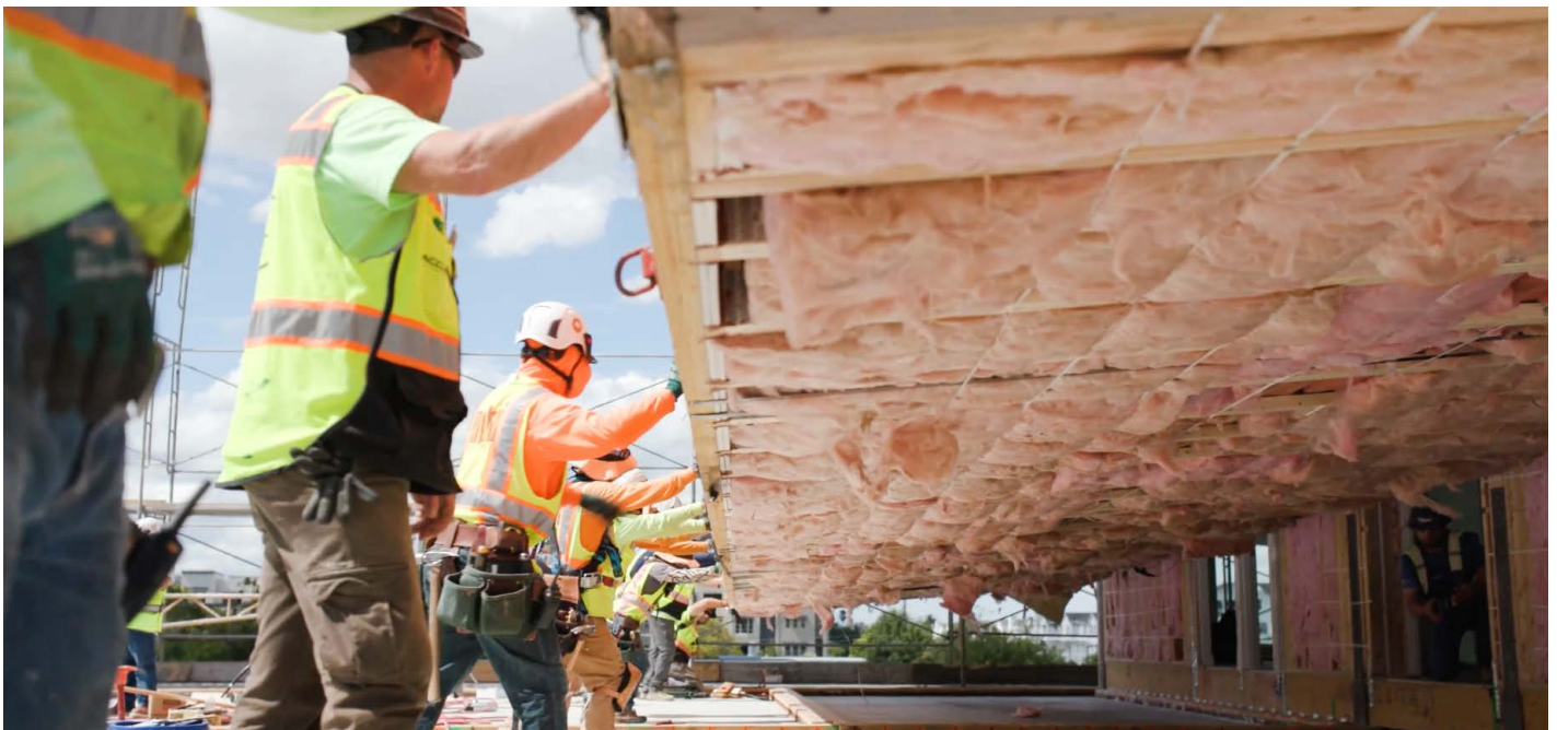
The Sango Court building was assembled over a 12-day period thanks to careful planning and expert consulting.
