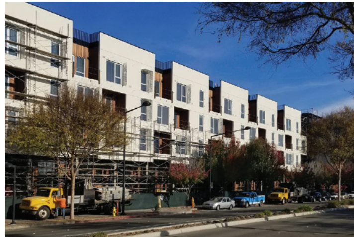
Erection of modular units to form a finished building
